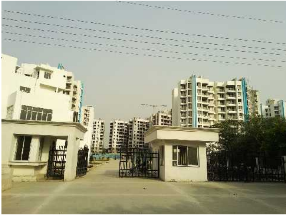
MAIN GATE & BOUNDARY WALL - 79.51 % WORK IS COMPLETED
