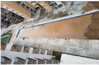
BALANCE AREA WATER PROOFING COMPLETED & SOIL FILLING IN PROGRESS
