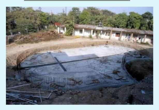
**SWIMMING POOL – (OVER ALL COMPLETION = 19.50%)**RCC OF RAFT 70% COMPLETED
