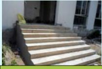
FIXING OF KOTA STONE AT STAIRCASE
