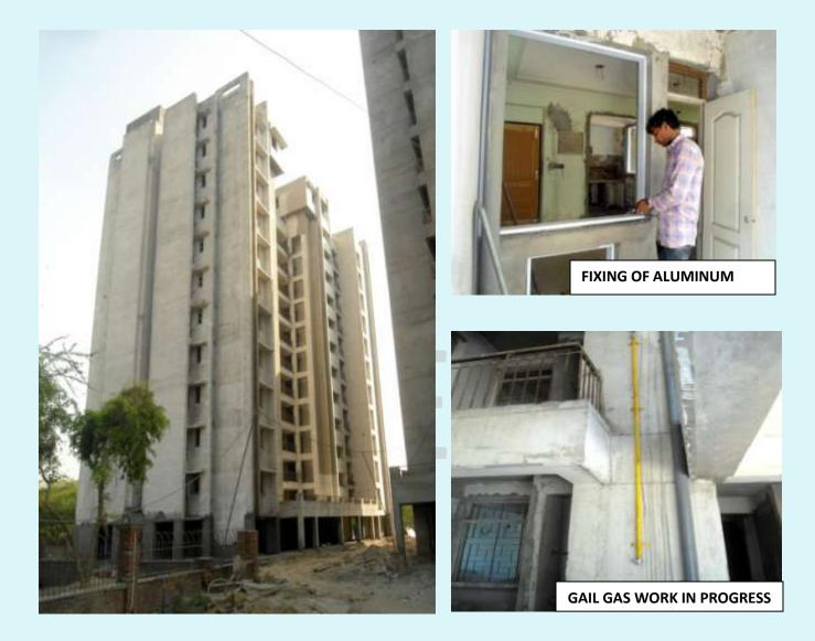
TOWER- 8 (TYPE B-1 & TYPE B2) Total Floor – Stilt + 11 Total flat = 33. Progress – Fixing of main frame of aluminium in widows & Gail Gas pipe line work. Overall completion 87.00 %
