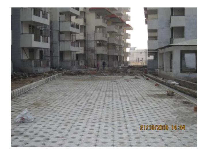
**PROGRESS:** Overall 25% area development over Non-Tower Area upper basement roof has been achieved. Those works are like roof top water proofing, filling of earth and laying of fire fighting path are in progress.
