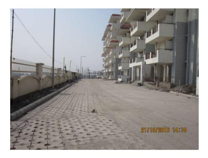
**PROGRESS:** Overall 90% area development work on south side has been achieved. Works are like laying of Concrete road, paver blocks upto gate no. 02, sewer/drain line connected up STP, external fire fighting line, HDPE water line has been completed.
