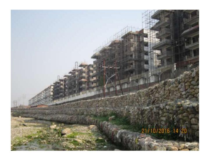
Gabion wall constructed adjacent to north side boundary wall in 31 May 16 to prevent flooding and soil erosion.
