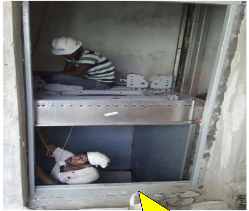
LIFT CABIN FIXING
