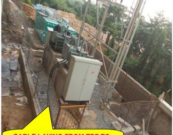
CABLE LAYING FROM TRF TO PANEL AT S/S-2
